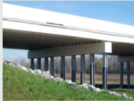
Prestressed box beams
