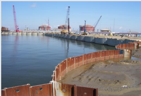
Flat web steel sheet pile
