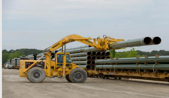
Coating Facility, Birmingham, AL
