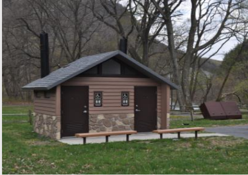
Precast concrete building
