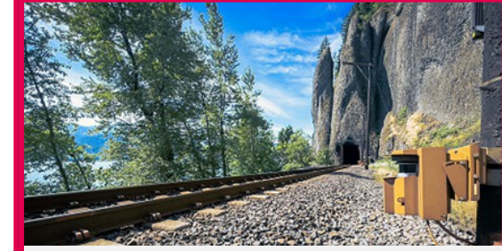
Wayside technology to detect rockfall, flood, and other dangerous conditions
