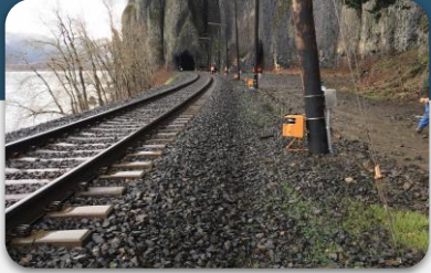
Rockfall Monitoring System
