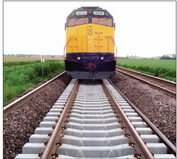
Heavy haul track construction using CXT® Concrete Ties.
