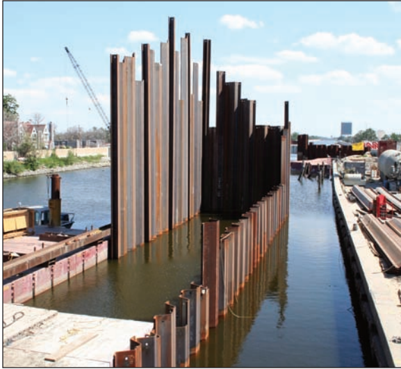
Steel sheet piles driven in a foundation construction project.
