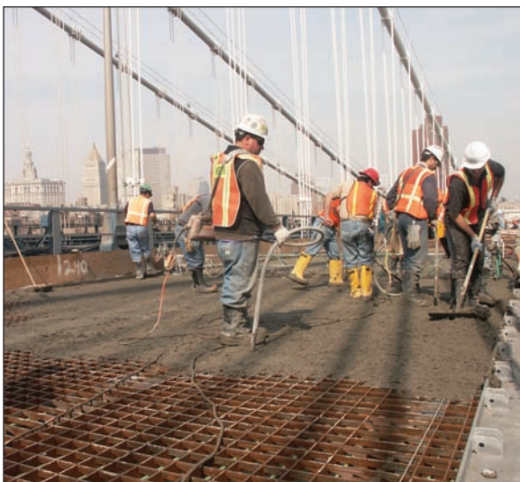
Steel grid decking installed on a bridge rehabilitation project.
