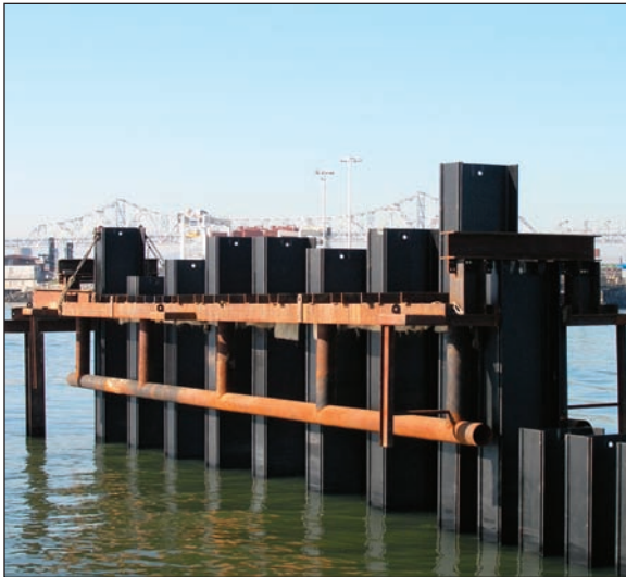
Engineered Combi-Wall for a harbor containment structure.
