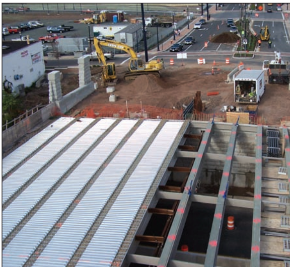
Structural steel stringer beams fabricated for a bridge renovation.
