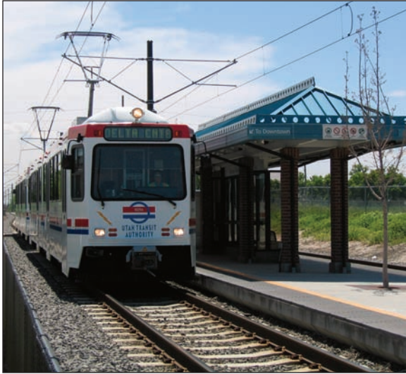
New welded rail and CXT® Concrete Ties for a commuter line.
