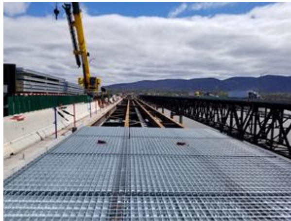
L.B. Foster manufactured steel grid bridge deck panels being installed on North Span of Newburgh-Beacon Bridge
